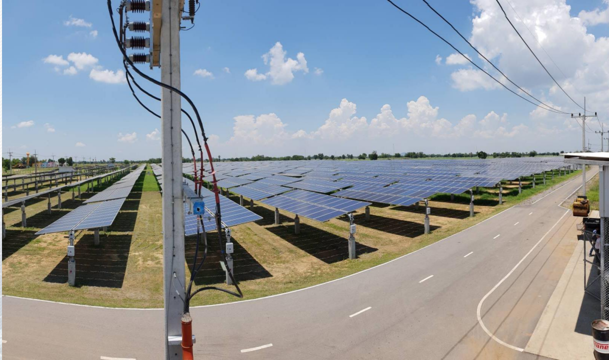
ACTUAL PHOTO FROM SITE VISIT
